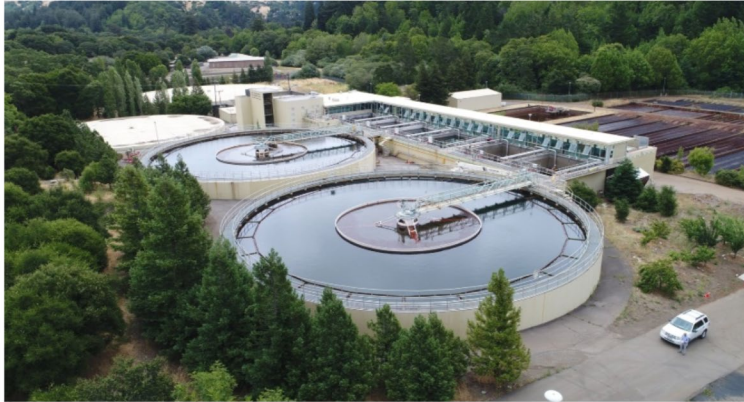
Seismic Upgrades to Clarifiers ($20M)
