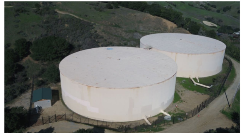
Rehabilitate Smith Saddle Tanks ($7M)
